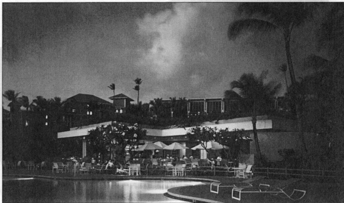
The design-build renovation and expansion of the Kapalua Bay Hotel in Maui was completed in mid August.
