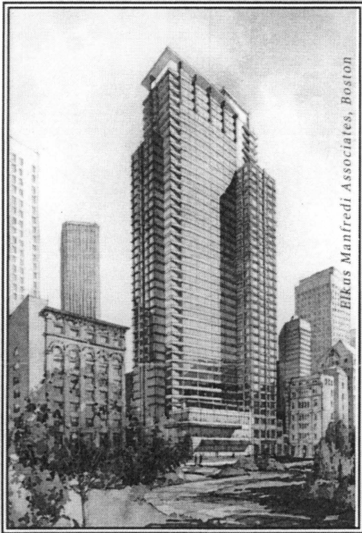
The 39-story 3rd & Mission Apartments, has generated articles in Engineering News-Record (June 14, '99) and the Wall Street Journal (July 7, 1999) for its record-setting concrete height in seismic zone 4.
