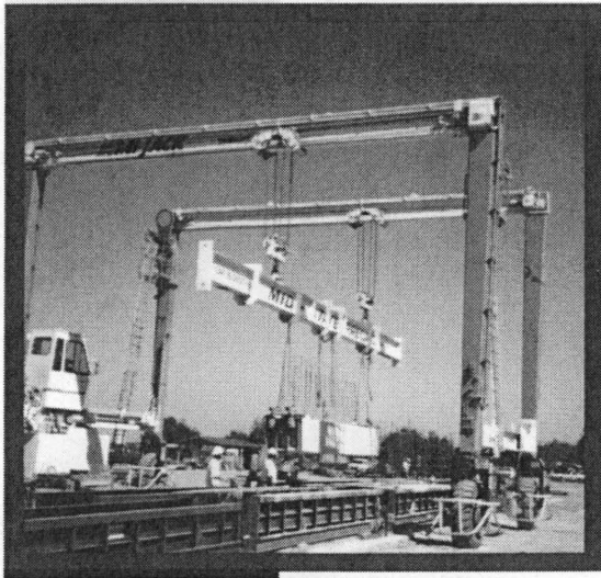
Mi-Jack removing beam from form at Mid-State Precast.
