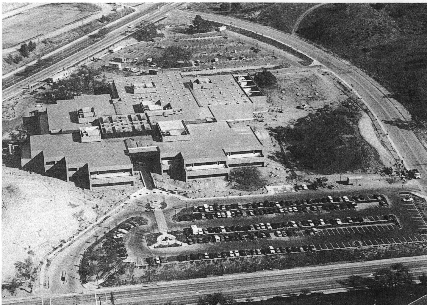
GTE Headquarters nearing completion
