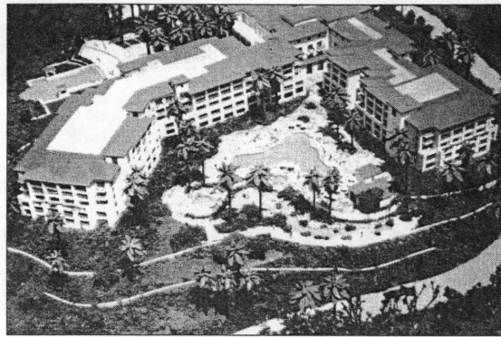
A portion of Four Seasons Resort Aviara's main hotel building which includes 320 rooms.
