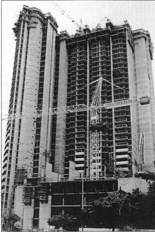
Park Place under construction
