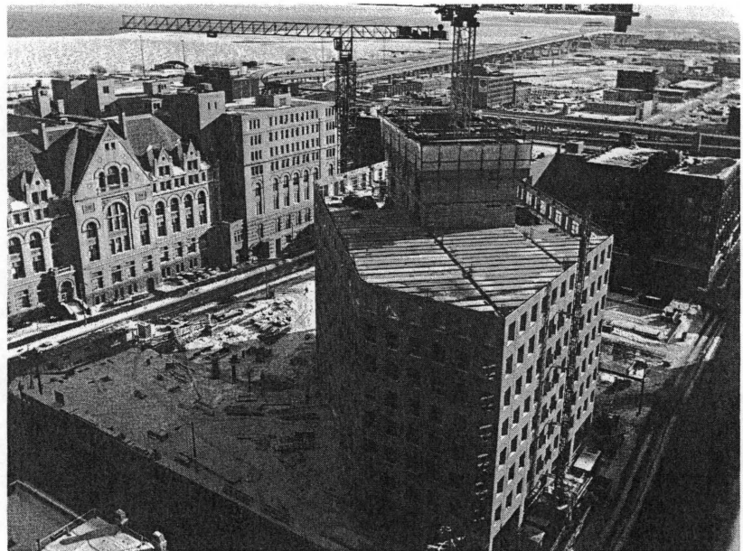
411 East Wisconsin Building
