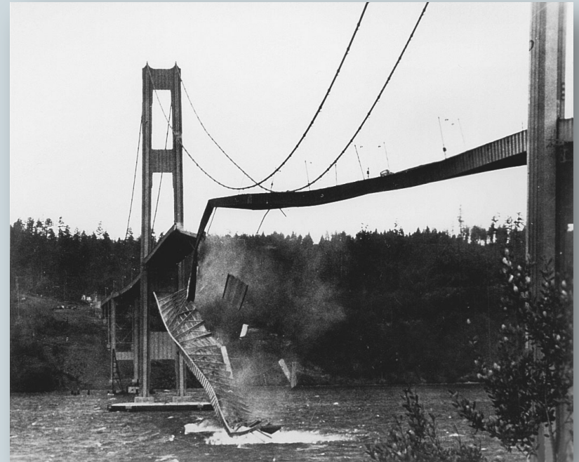
Tacoma Narrows Suspension Bridge “Galloping Gertie”
